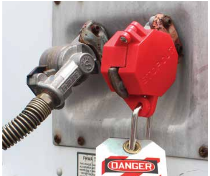
Secure with padlock and tag.
