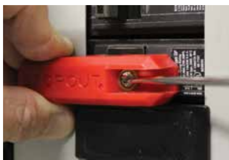
Tighten setscrew for secure fit.
